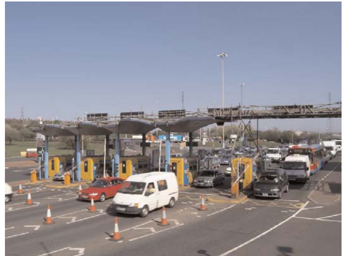
The Automatic Toll Booths at the Tunnel
